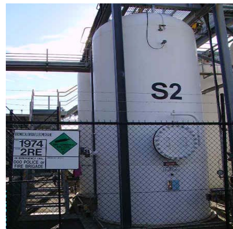
Halon Bank Bulk Storage Halon 1301.
